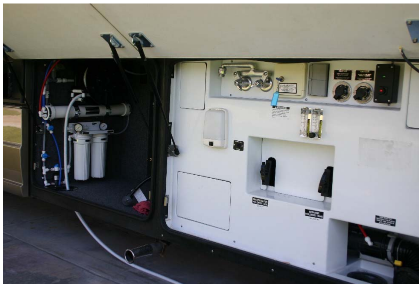
AUTOMATIC SYSTEM IN COUNTRY COACH MAGNA 630 GLENDINNING HOSE REEL, CONTROL BOX AND FLOW METERS ARE SHOWN
