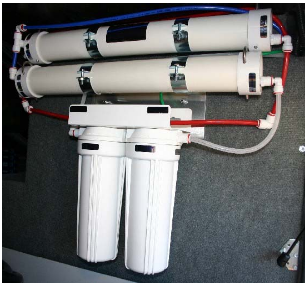
DOUBLE MEMBRANE SYSTEM INSTALLED IN THE TRAVEL SUPREME TWO MEMBRANES DOUBLE PRODUCTION WITHOUT AN INCREASE OF WASTE WATER
