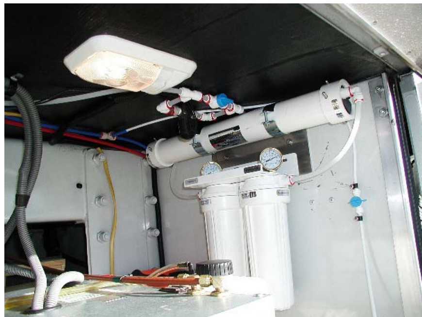
INSTALLATION IN ALPINE HYDROHOT BAY
